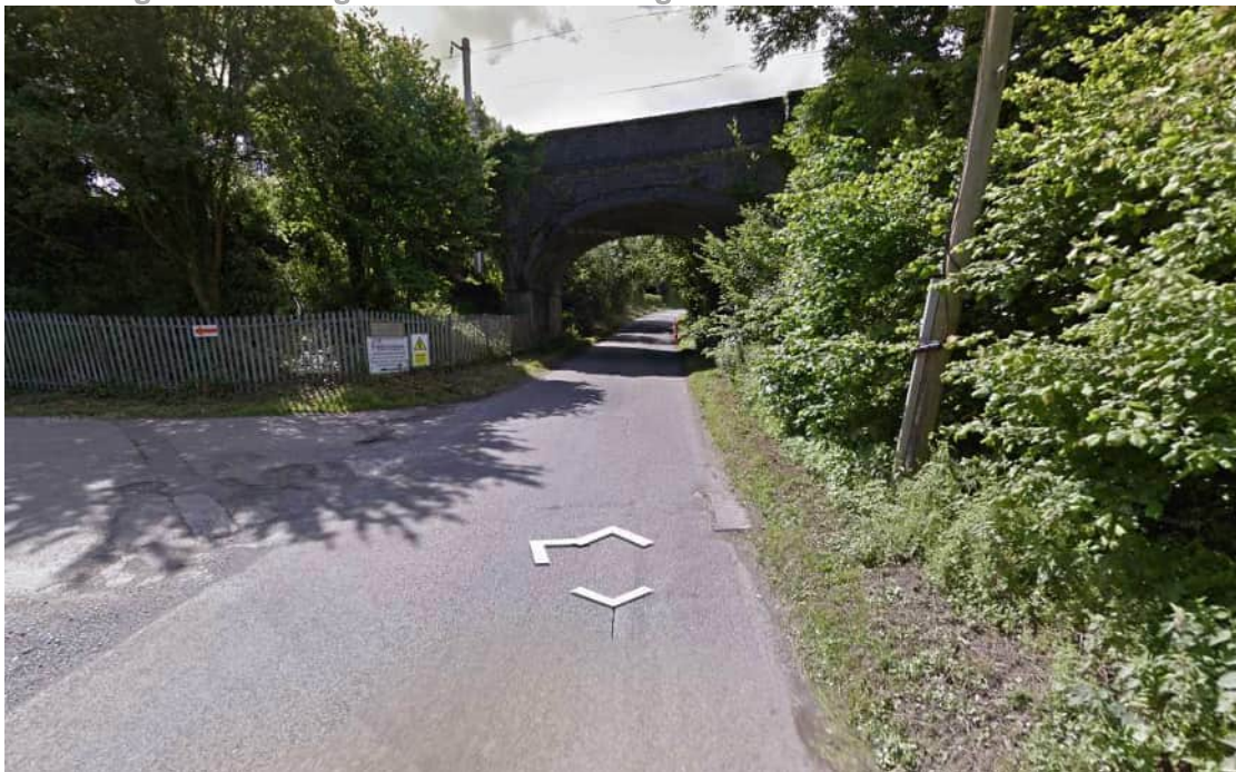
Fosse Way rail bridge (restrictions unknown)
